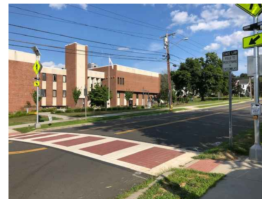
STAMPED BITUMINOUS CONCRETE CROSS WALK AT DEER HILL AVE. & CITY HALL
