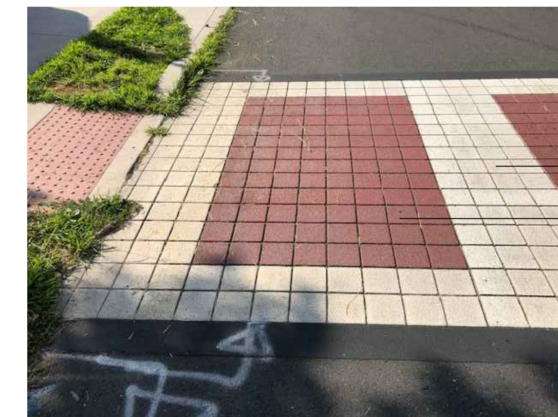
STAMPED BITUMINOUS CONCRETE CROSS WALK AT DEER HILL AVE. & CITY HALL
