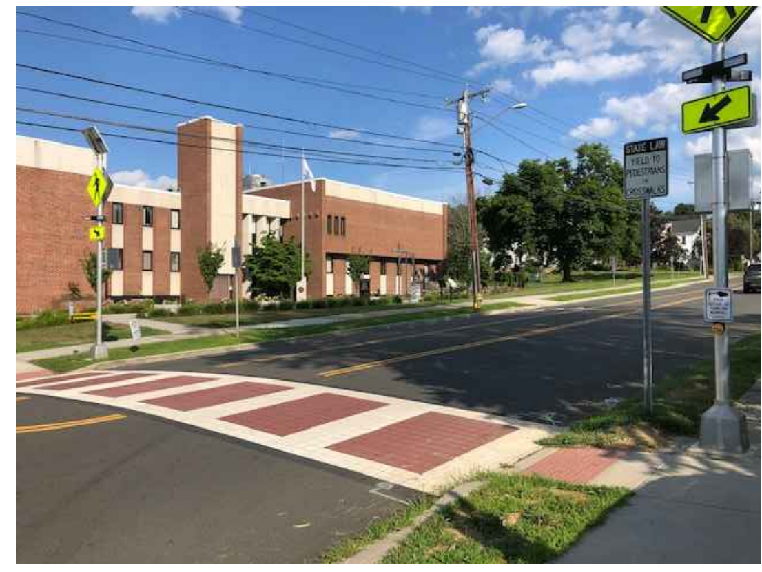
STAMPED BITUMINOUS CONCRETE CROSS WALK AT DEER HILL AVE. & CITY HALL NTS
