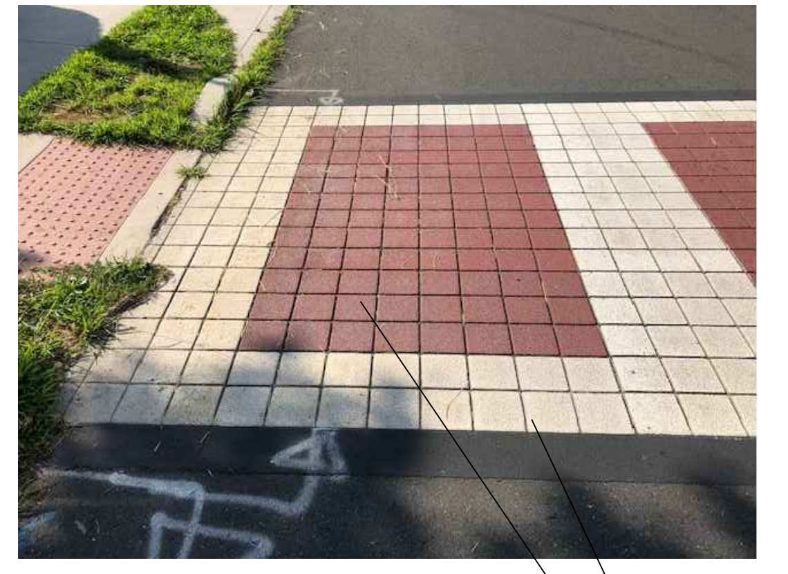
STAMPED BITUMINOUS CONCRETE CROSS WALK AT DEER HILL AVE. & CITY HALL NTS
